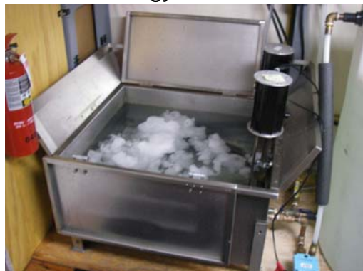
A snow melter is used to obtain fresh water at some Antarctic research stations
