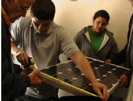
Students measuring the solar panel they will install on the rooftop canopy of their school's electric golf cart.
